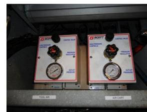
To utilize these systems, simply open the control valve and adjust the regulator to the desired position. At the conclusion, be sure to close the control valve and decrease the regulator to 0 psi.
